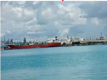
Seawater withdrawal point
